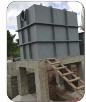
EQUIPMENT INSTALLATION PROCESS
