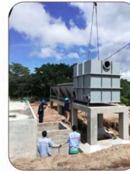
EQUIPMENT INSTALLATION PROCESS
