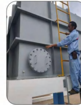
EQUIPMENT INSTALLATION PROCESS
